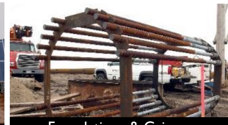
Foundations & Caissons and Directional Boring
